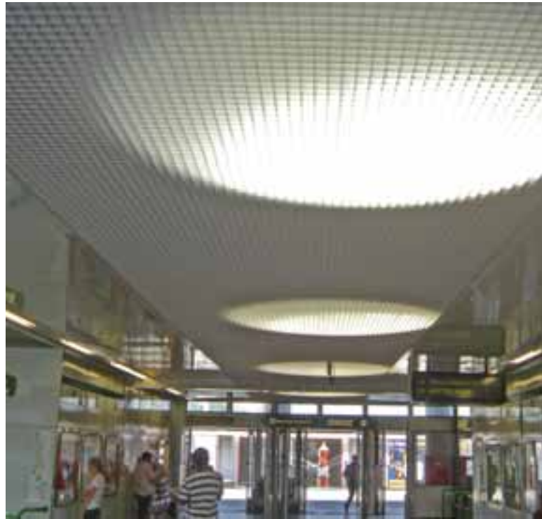
Underground station in Vienna, Austria, Aluminium with cell 50x50x50 mm
